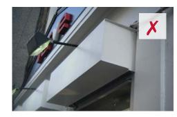
Roller shutters of the non-solid type may be acceptable in a perforated, lattice, brick bond or open weave pattern. Shutters made up of interlocking clear polycarbonate sheets running externally to the glass may also be acceptable.
