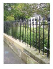
what the original railings were like. Remaining sections of iron work may still exist in the cope or on similar neighbouring properties or old photographs and plans can be used. In most cases, cast iron railings fixed individually into the cope should be used.
