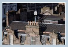
These satellite dishes are positioned in a roof valley and are not visible from street level. Fixed to later service features, they do not damage architectural details. © N. Haynes.
