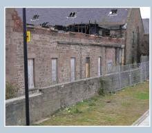
Former Arctic Tannery and Harbour Workshops, Dundee. A fire destroyed the upper part that had originally been of timber louvres to cure sealskin hides, replaced in brick. The development of housing (see below) echoes in a new form the timber and brick previously used here.
