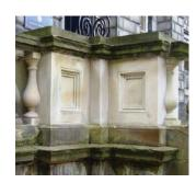
Where indenting is appropriate, the indent should be selected to closely match the original stone. Artificial stone should not be used on listed buildings.
