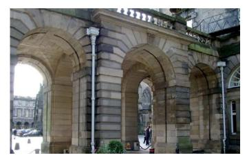
Replacement rainwater goods should match the original, cast iron or zinc should be used where these were the original materials. Other materials such as aluminium may be acceptable, where appropriate.
