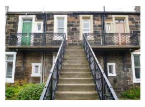
They are constructed of squared rubble with rustic quoins, raised margins to openings, slated roofs and pedimented gables. The external stairs are embellished with decorative geometric-patterned ironwork handrails to steps and balconies.
