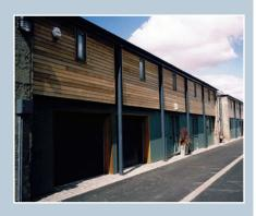
Complementary: Dundas Home Farm, South Queensferry, an 1881 steading converted and extended for residential use from 2001 to 2006. Here a new range takes its cue from the scale and rhythm of the original. © Simpson & Brown Architects.
