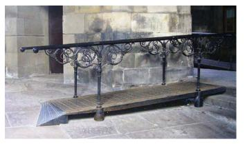
Where appropriate, consideration should be given to regrading the ground at the entrance in order to overcome the need for larger ramps and minimise the visual impact on the building. If this will cause a footway hazard, a ramp inside the building may be appropriate; the removal of steps and the lengthening of doors can sometimes accommodate this.
